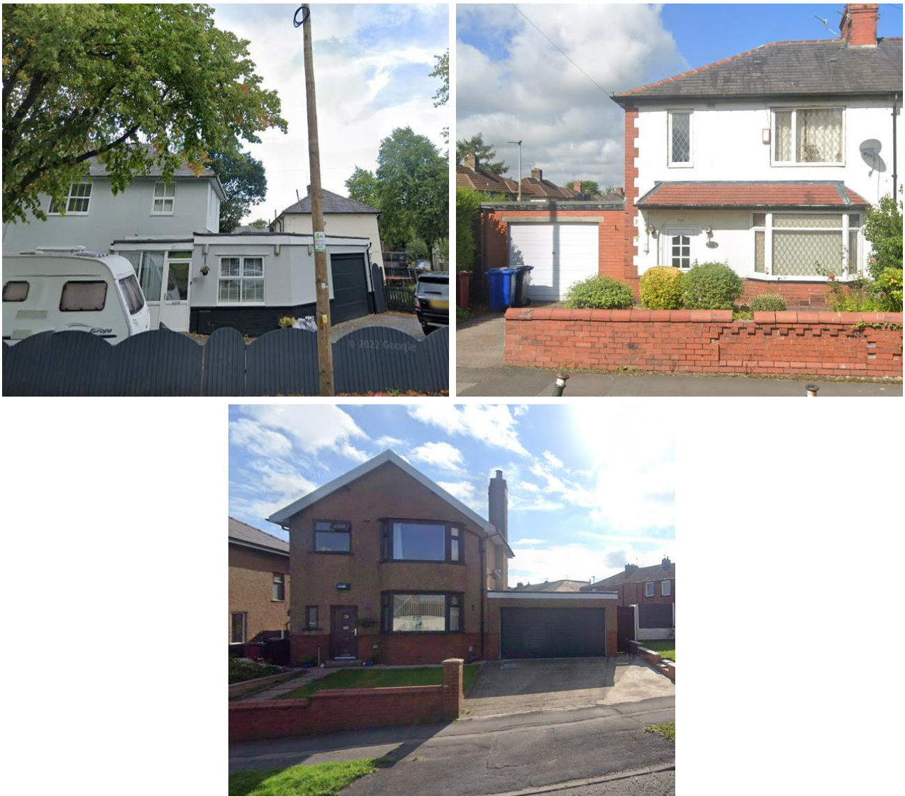
Figure 4: Existing Flat Roof Side Extensions (Left Top – 77 Green Lane, Right Top – 106 Shorrock Lane, Middle Bottom – 221 Shorrock Lane)
