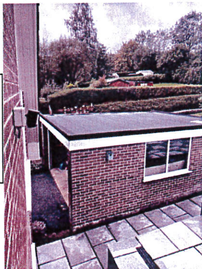
View from the patio doors at the application site in to No.71 Manor Road.
